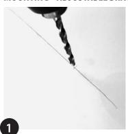
Check product orientation. Mark hole positions from brackets pre installed on MOMO-L base (2 per metre/40") and drill if required.
